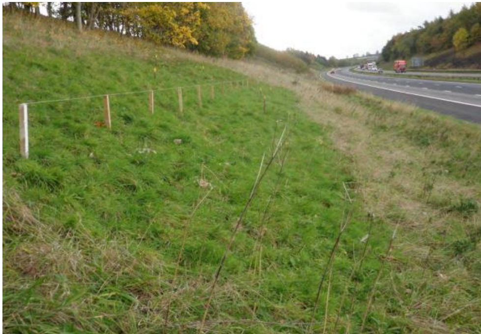
Figure 23: View of the site looking southeast prior to the installation of the willow poles. The peg line defines the back scarp and the toe bulge is also visible (from EM Highways 2014)
