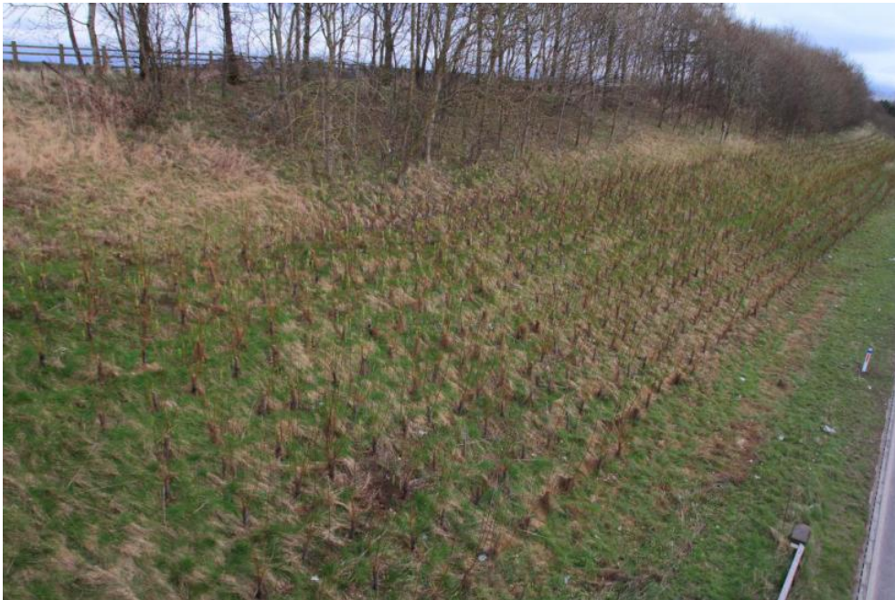
Figure 24: General view of the M6 south of J40 site from the B5320 overbridge looking south-east (Site Photograph 7DW_4242)
