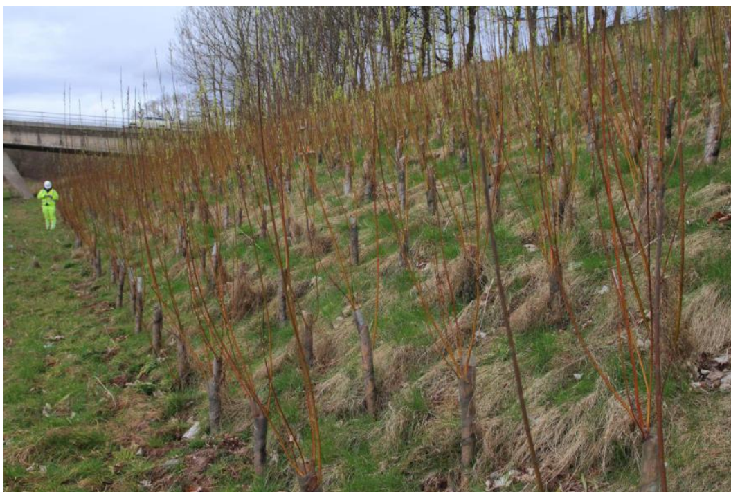
Figure 25: M6 south of J40, view of toe of slope looking approximately north-west towards the B5320 overbridge. The toe bulge is more discernible in this image (Site Photograph 7DW_4256)
