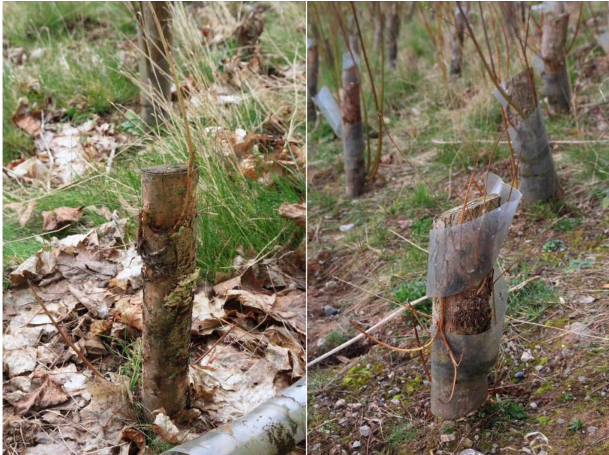
Figure 27: M6 south of J40. Growth of mould/fungi on willow poles (left) and the translucent plastic wraps used to protect the poles and shoots from animals (right) (Site Photographs 7DW_4260 [left] and 7DW_4258 [right])
